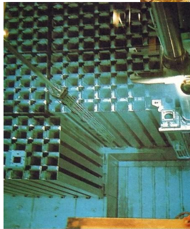
Ringhals PWR Storage Racks
